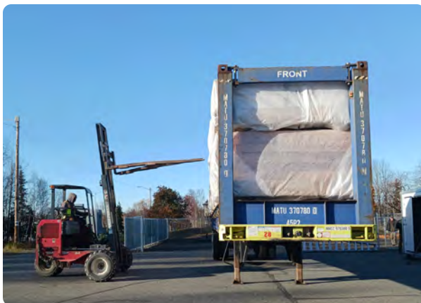
A worker delivers SIPs materials to the site, October 2024.
