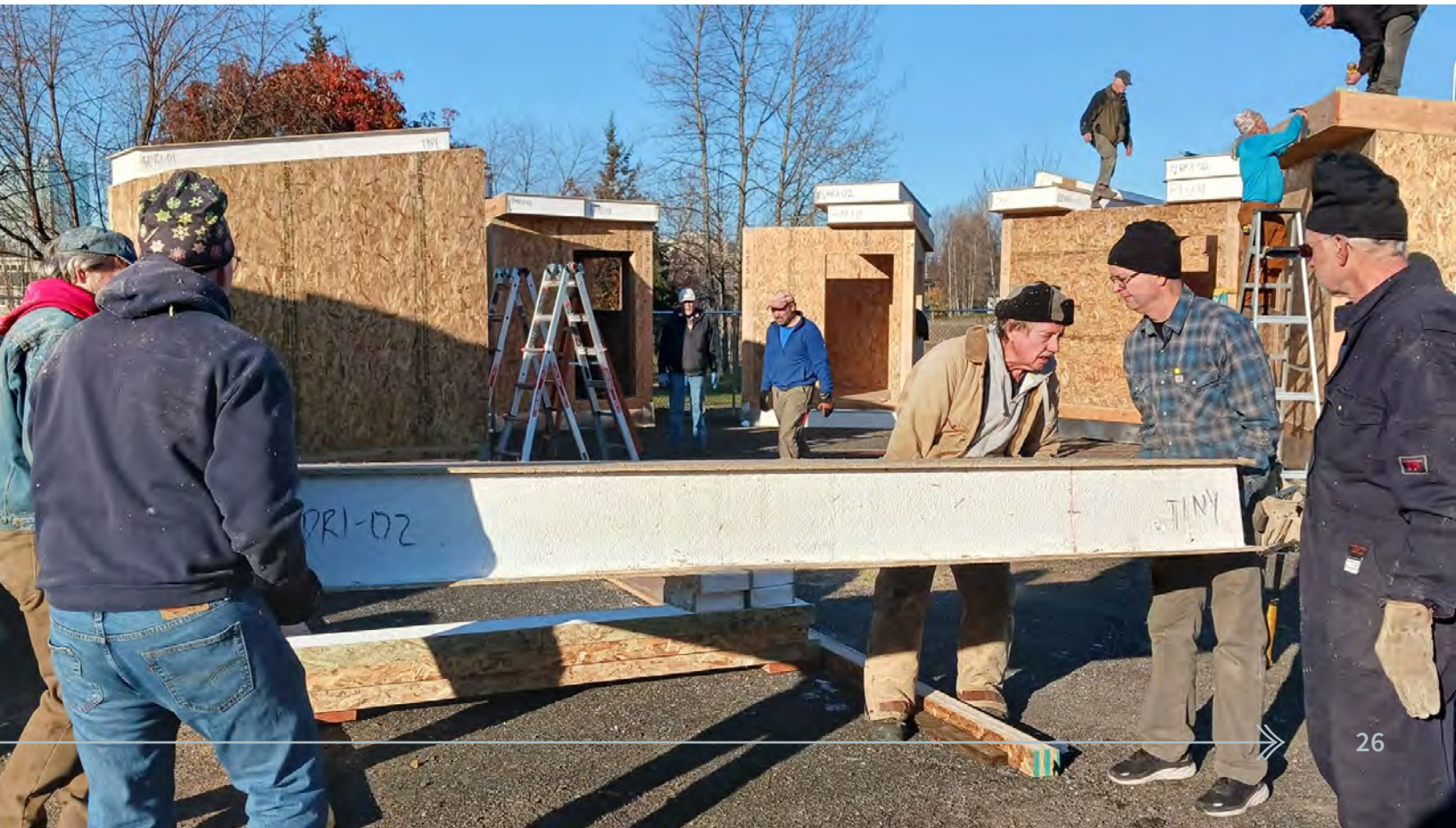
Volunteers build the cabins, October 2024.
