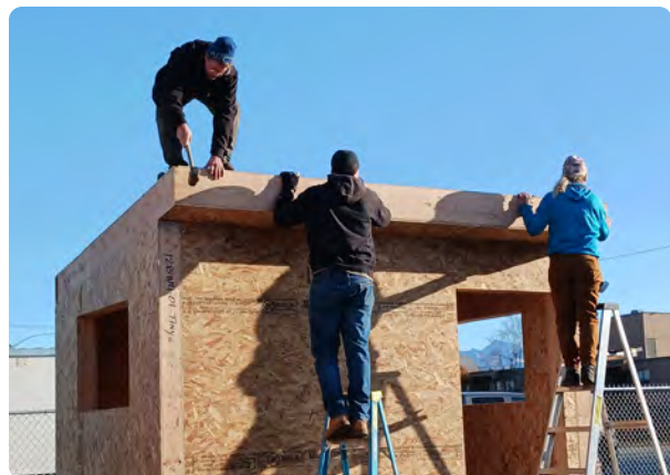
Volunteers construct the shelters, October 2024.
