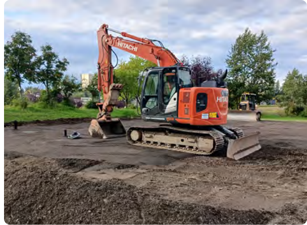
Site excavation and leveling begins, September 2024.
